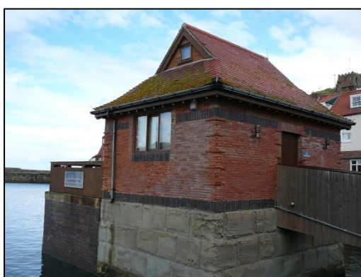
Former Sewage Pumping Station
